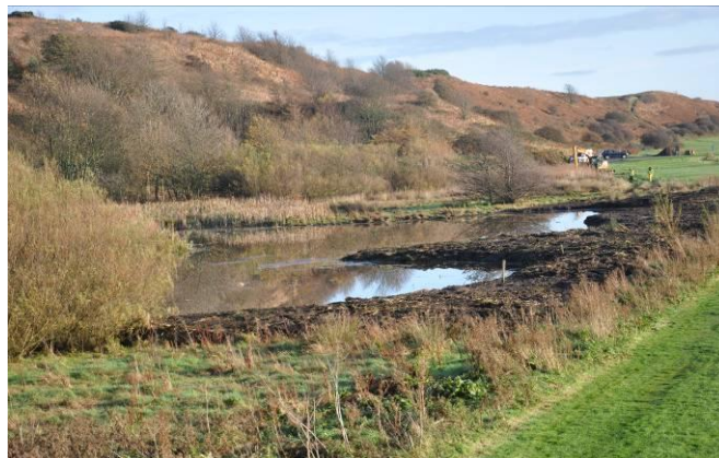
First stage nearing completion
